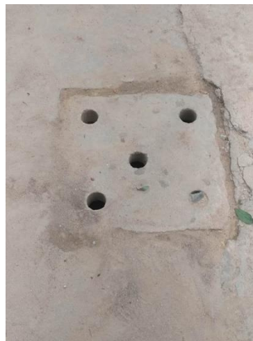
Figure 4-13: Rain water recharge pits
