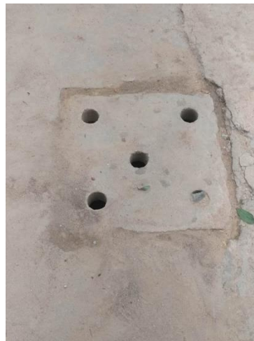
Figure 4-9: Rain water recharge pit
