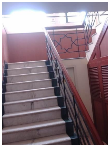
Figure 5-10: Well-ventilated and day-light integrated premises
